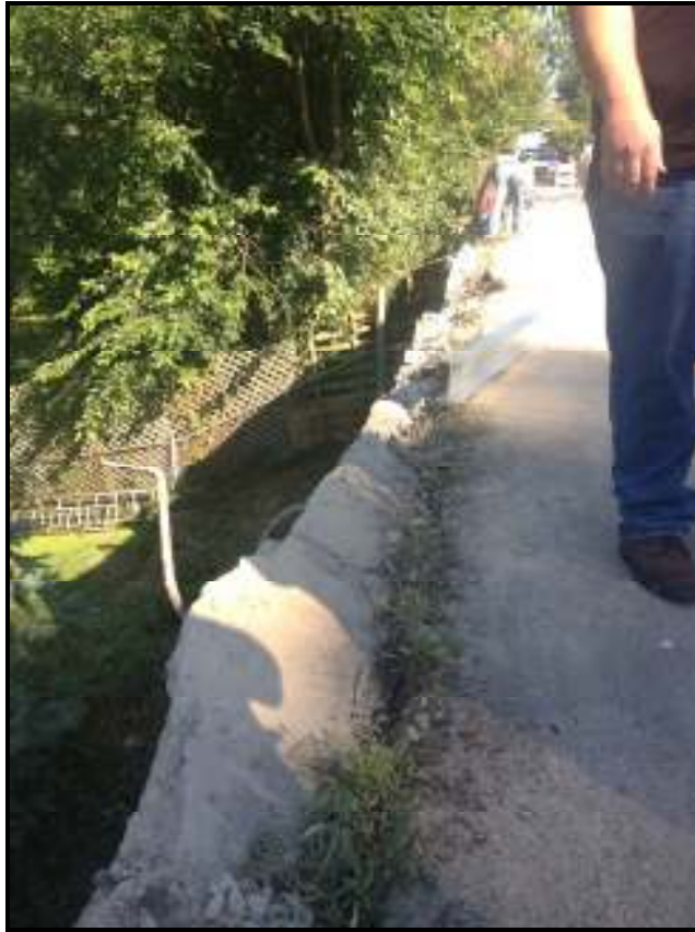
Photo of Demolition of Walkway on Kaufmann Avenue
