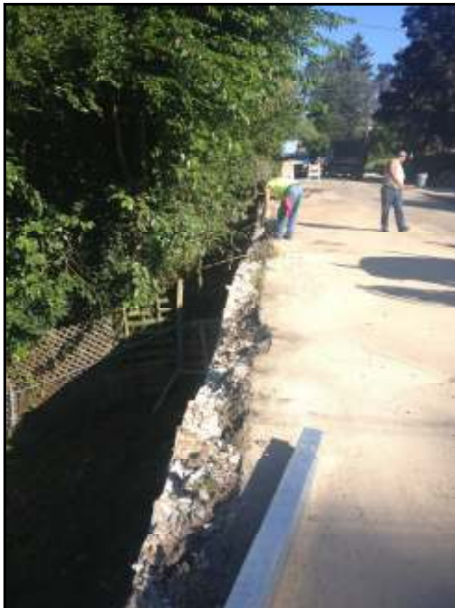
Photo of demolition of Cantilever Walkway on Kaufmann Avenue
